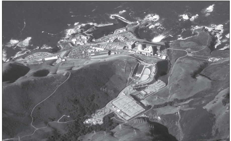
Diablo Canyon Nuclear Power Plant on the coast of California
